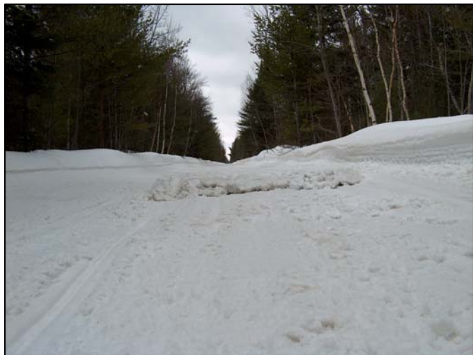
Photo 4.11 Don't leave a hazardous pile of snow in the trail when adjusting a drag
