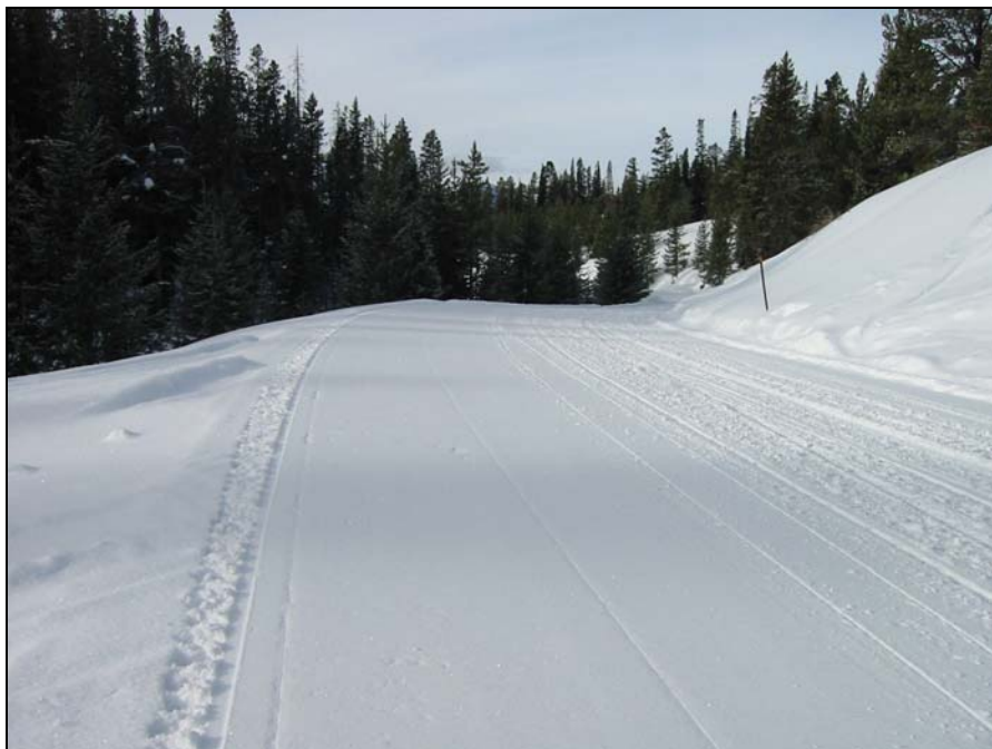
Photo 1.8 Trail grooming builds a solid, compacted base
