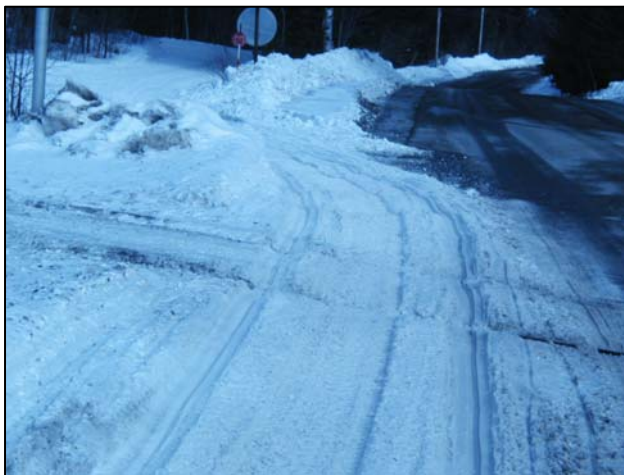
Photo 4.9 Use care to not create snow/ice buildup on railroad tracks
